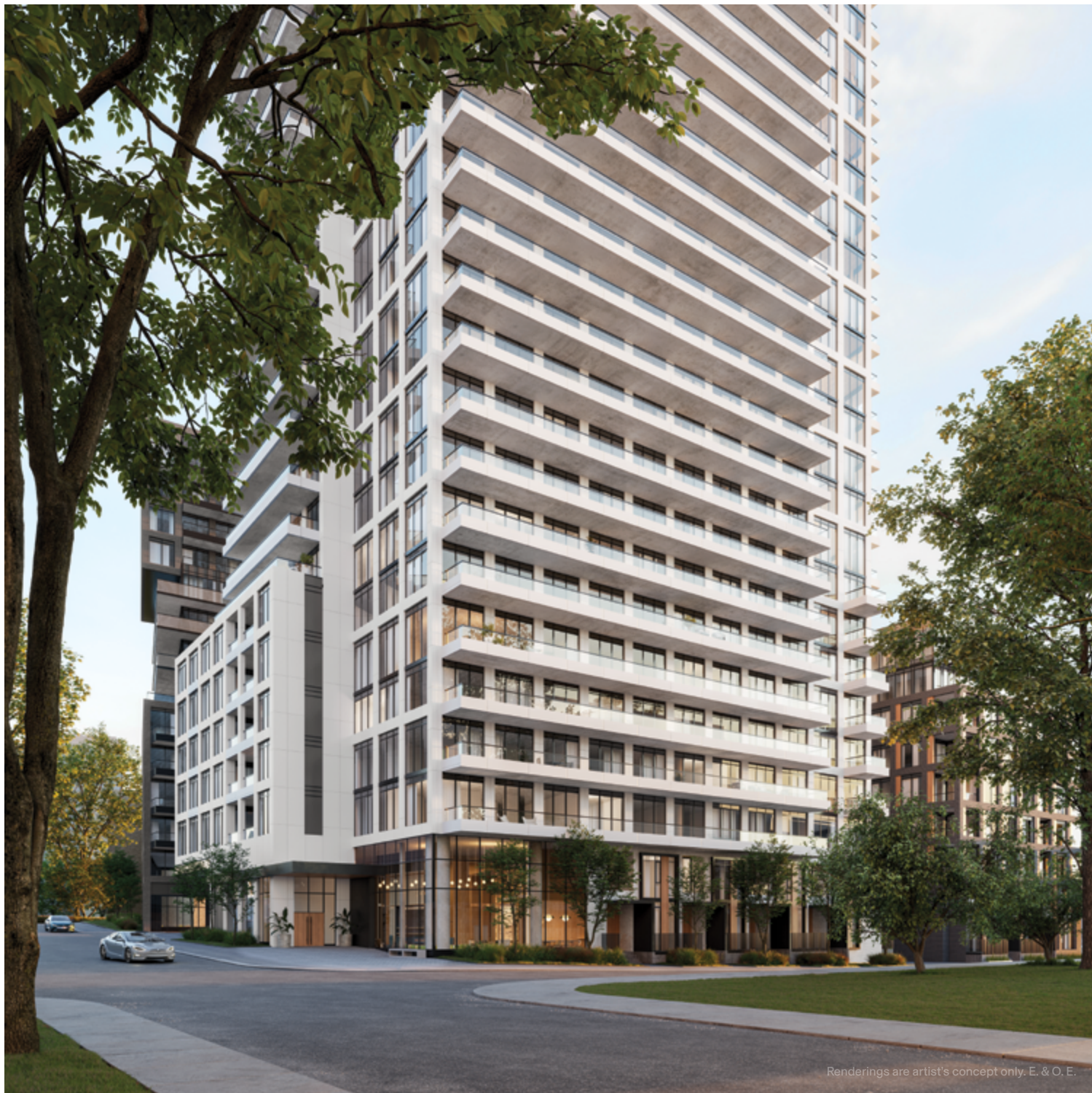
Above Corktown, Lobby Entrance
