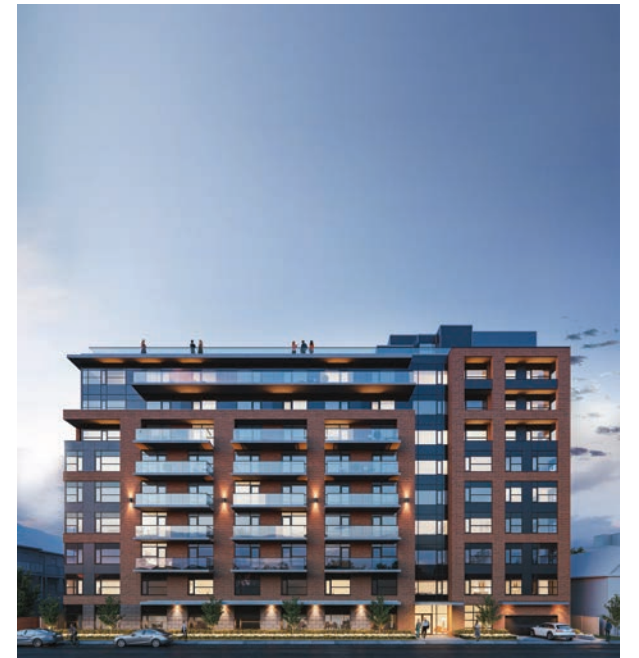
CAPITAL PARK Ottawa | 291 Units (Completed)
