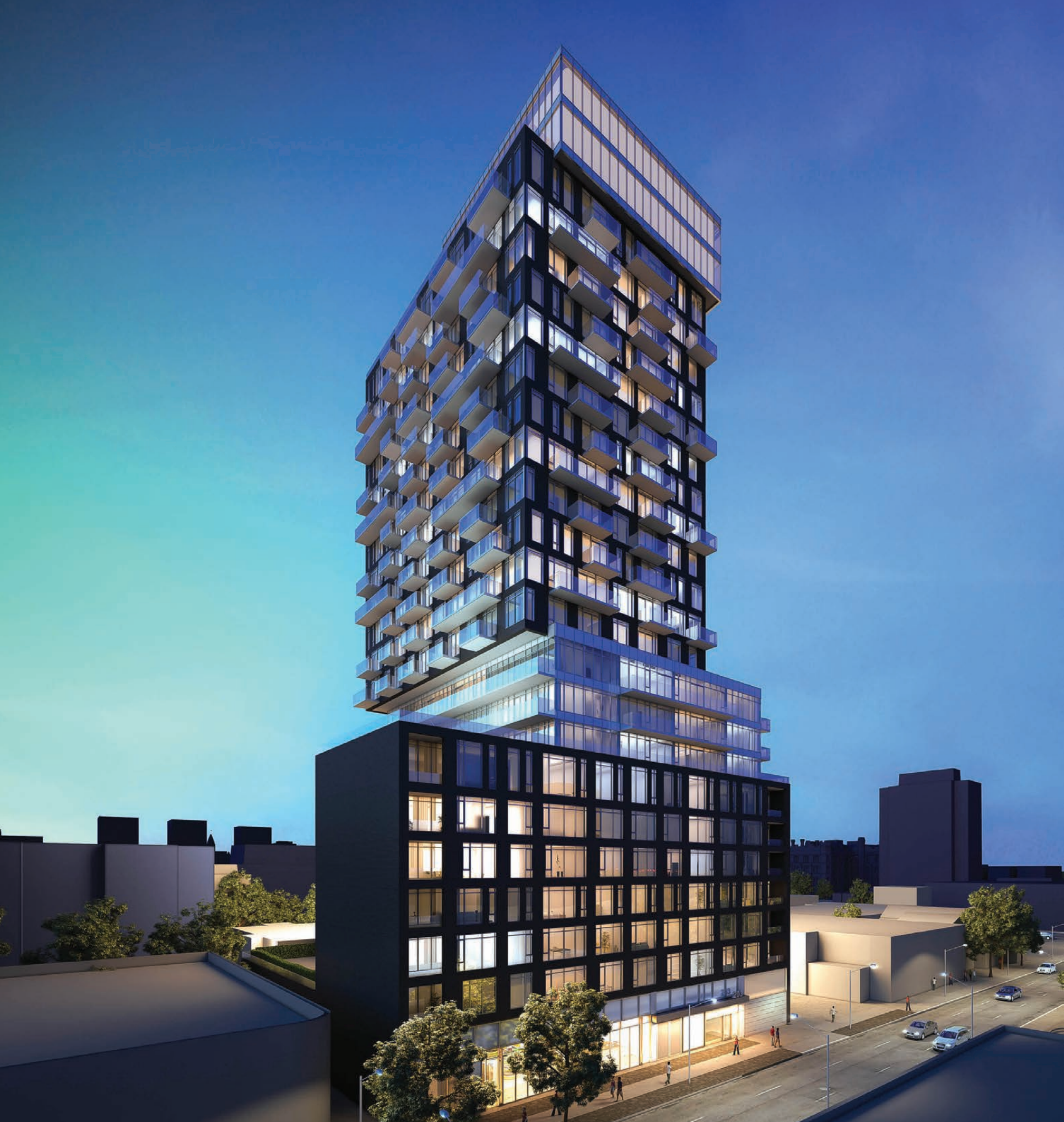
SOBA, OTTAWA COMPLETED 2019
