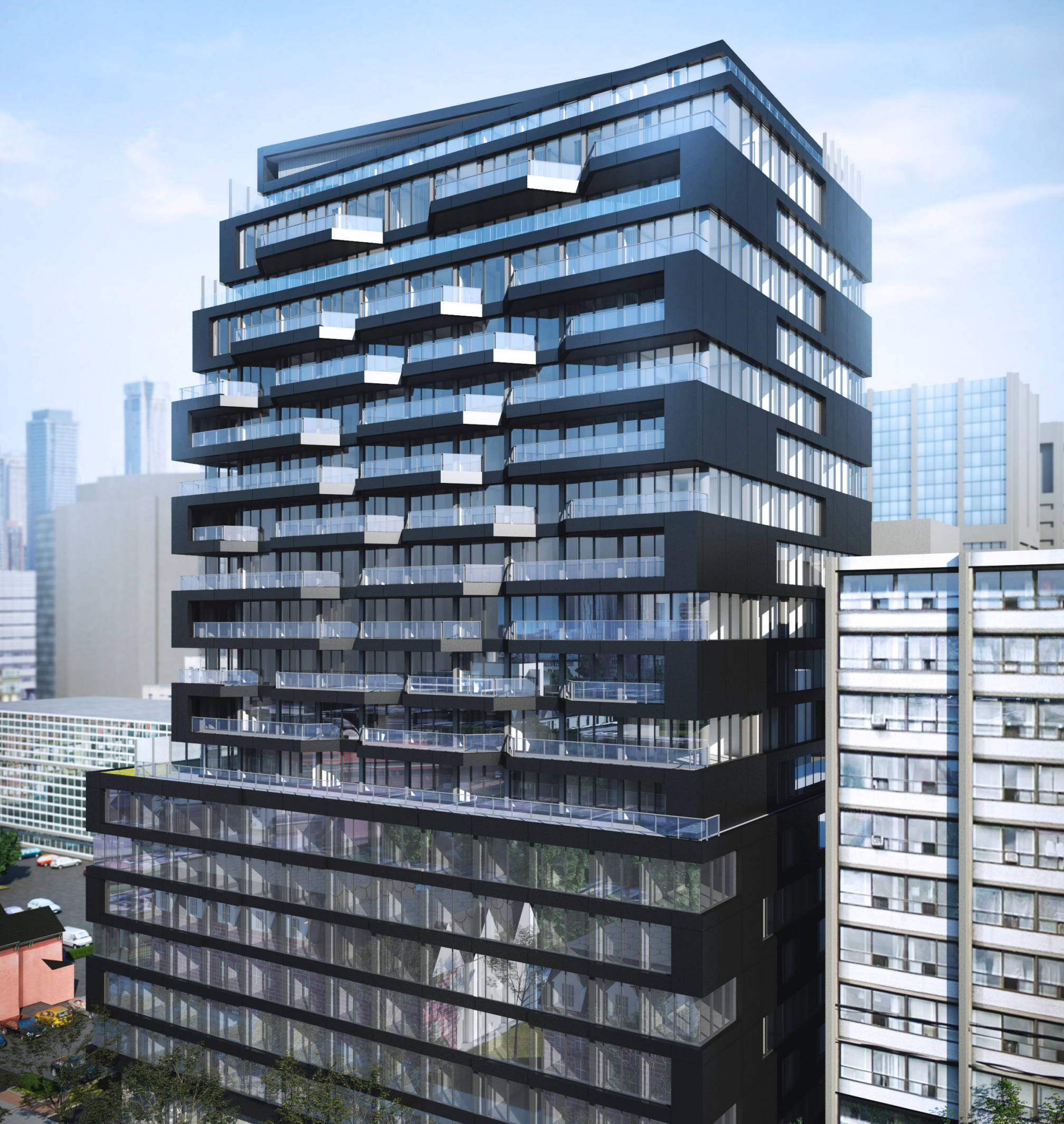
THE BREAD COMPANY, TORONTO UNDER CONSTRUCTION
