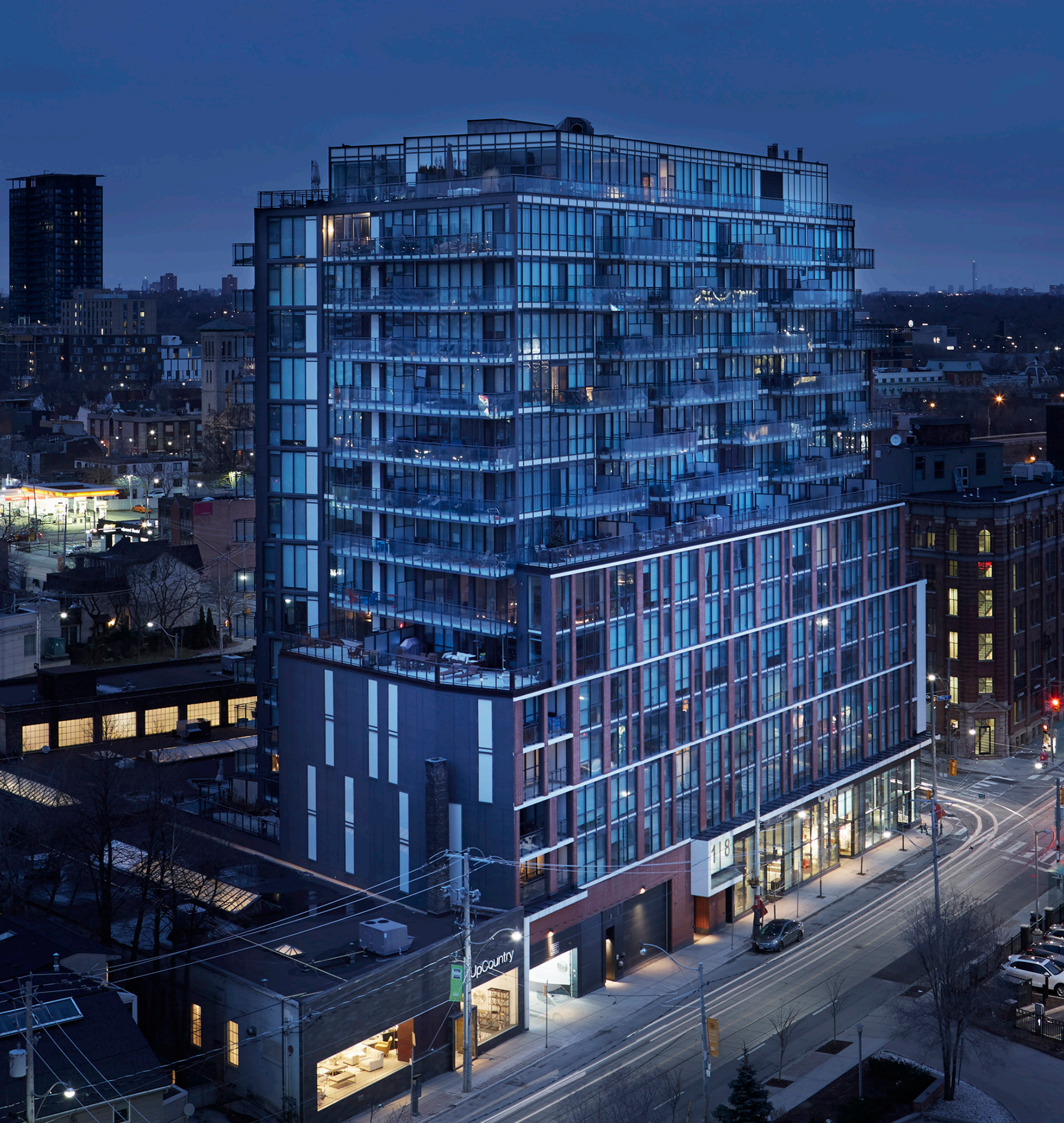
THE KING EAST, TORONTO COMPLETED 2012
