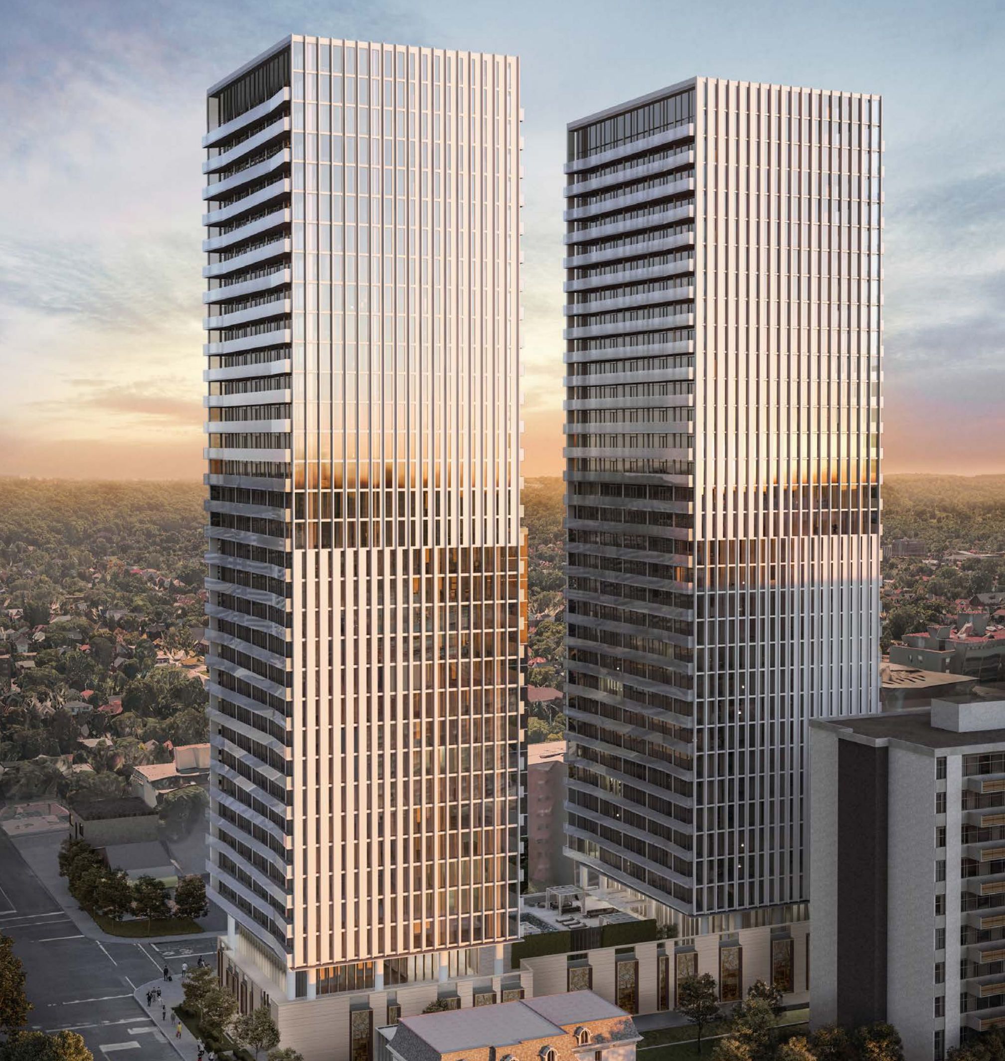
TELEVISION CITY, HAMILTON UNDER CONSTRUCTION
