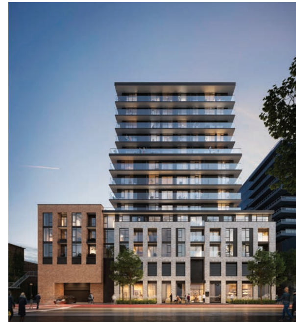
1 JARVIS Hamilton | 354 Units (Under Construction)
