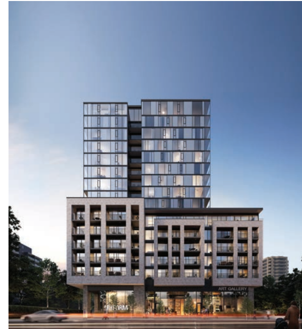
ARTFORM Mississauga | 336 Units (Under Construction)
